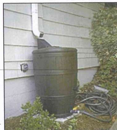
A rain barrel used to collect rooftop runoff using a gutter / downspout system
